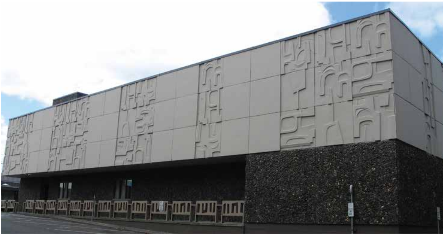
Sculpted relief panels created by James Lee Hansen for the “Land Title Building” (now iQ Credit Union), Vancouver, 1963, cast concrete, 15’ tall.
